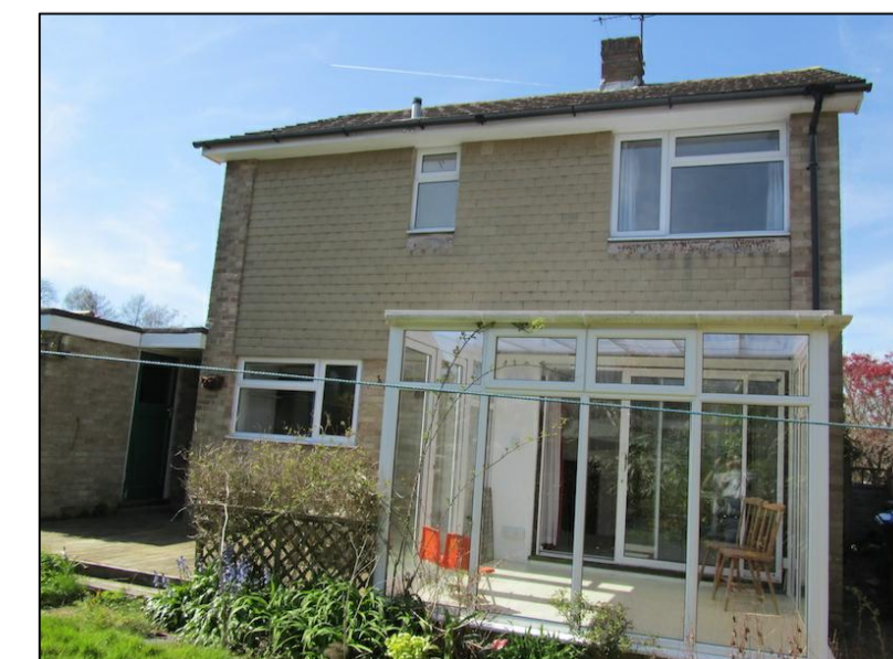
PHOTO SHOWING REAR OF EXISTING PROPERTY
